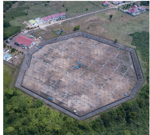
Equatorial Atmosphere Radar in West Sumatra, Indonesia. Its size is about the same as that of the MU radar.
